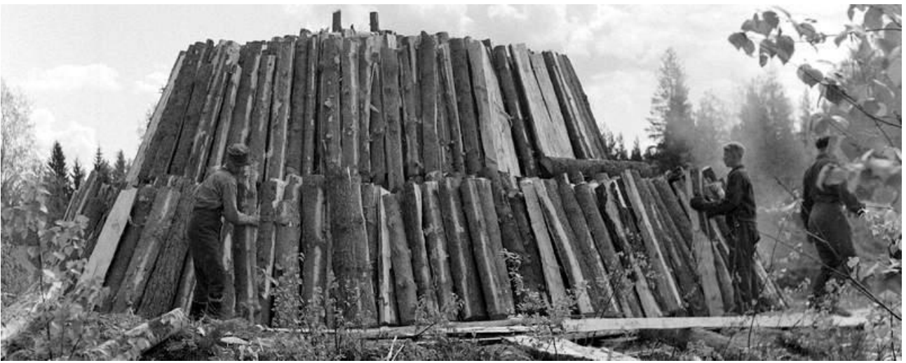
"Gasoline" for cars -factory - Coal burning wood-gas operated vehicles- Koksin valmistus puukaasuautoille.
